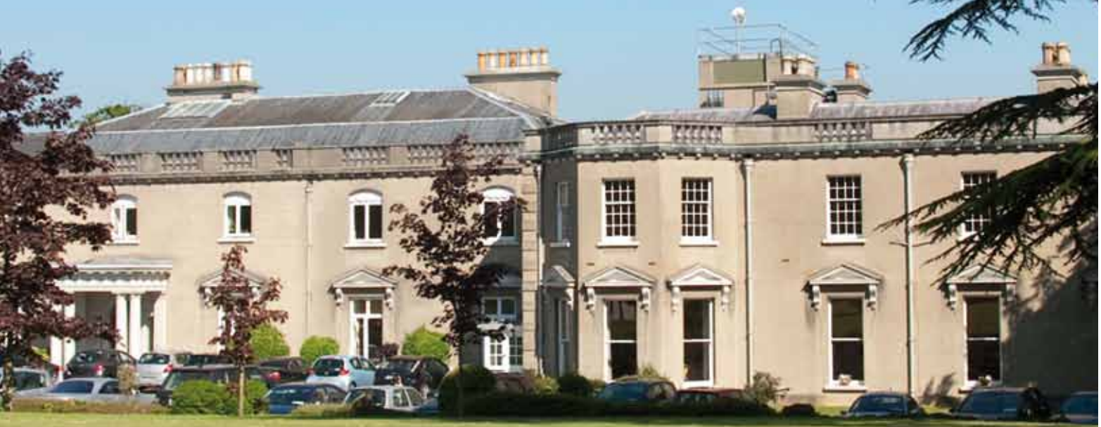
St Edmundsbury Hospital, Lucan, Co. Dublin
